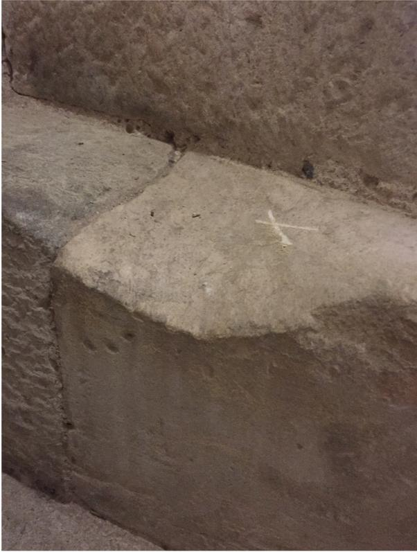
The tower stairs are over five hundred years old. Twelve of the steps were very worn and needed to be cut out by skilled stonemasons and replaced with new stone. We now have the funds thanks to GCG Environment Trust and work was completed in Spring 2021.
