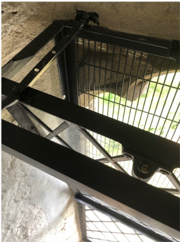
Close-up of the new opening mechanism, showing a range of positions to ventilate the chamber
